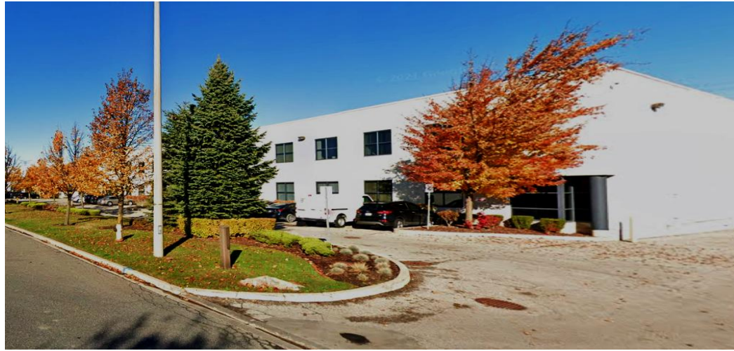
Image: Street view of a two storey office and warehouse building
