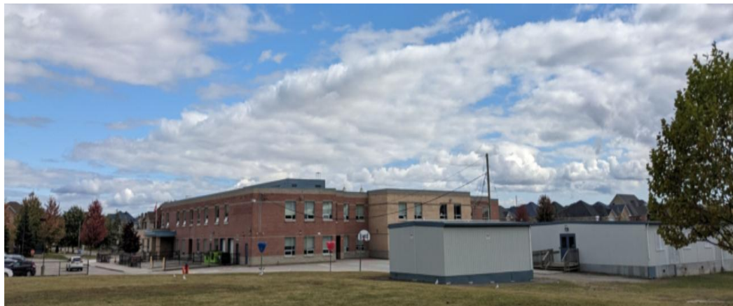
Image: An elementary school with portables
