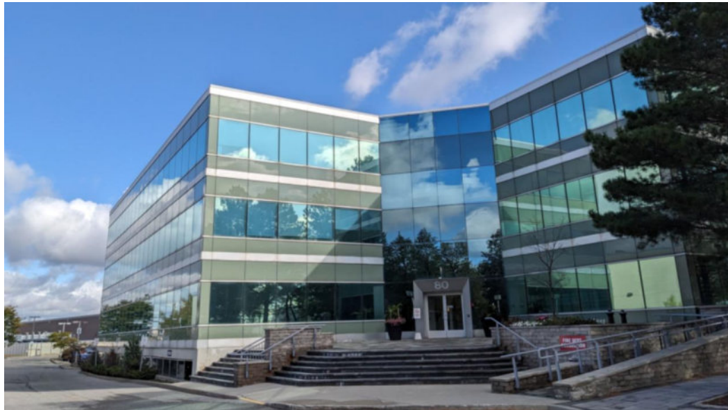
Image: A medium sized office building with large spandrel glass windows
