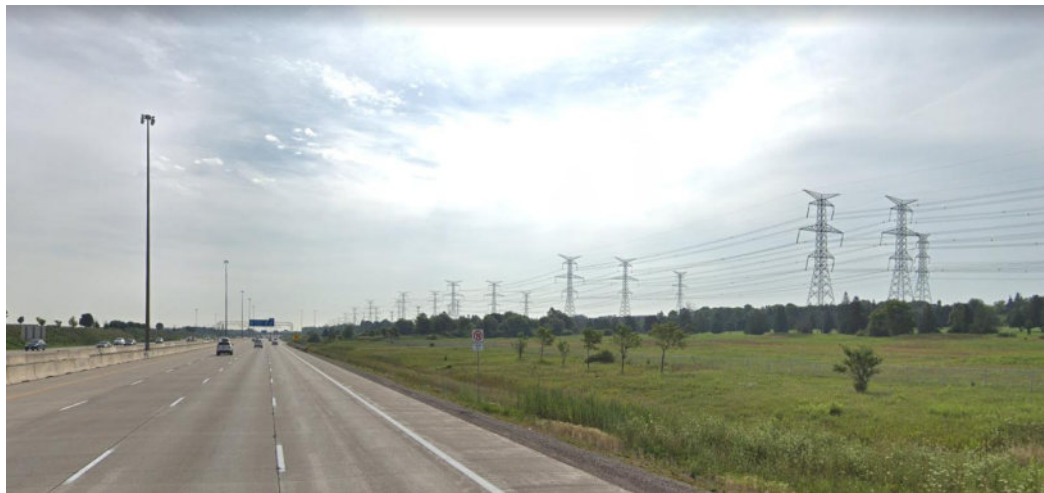
Image: Highway 407 and hydro corridor
