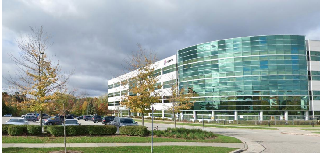
Image: A large multi-storey office building with curvilinear spandrel glass wall
